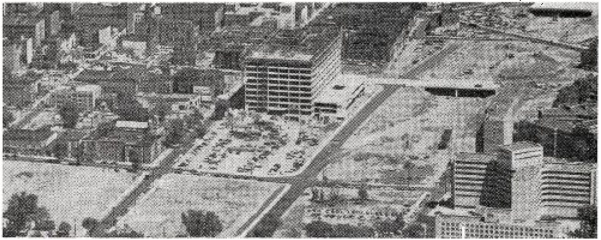
New Haven's new look • Downtown slums razed to make way for modern buildings and trough scooped for new expressway. Southern New England Telephone this fall will move 2,500 employees into new plant (center). Several redevelopment projects are in works.
